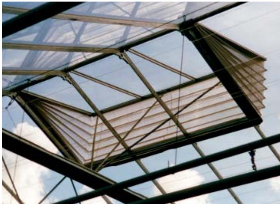
Photo 1. Insect screen fitted to a ventilator in a Venlo glasshouse. The screen is manufactured to have a concertina shape which unfolds as the ventilator opens.
