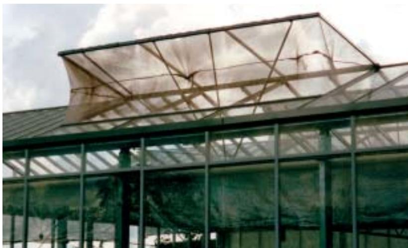
Photo 2. An insect screen fitted to a roof ventilator. The distortions formed where the five strings that prevent the net from billowing outwards are attached to the reinforcing strip half way up the screen can be seen.
